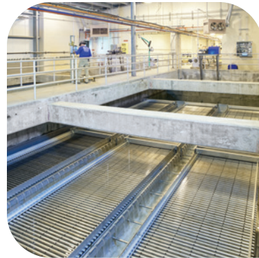
↑ MRI's break-down style cartridges, optimal for confined installations
