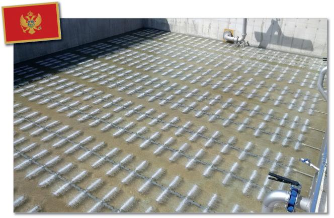
OTT aeration system based on MAGNUM® FLEXNORM® membranes and AirRex® piping system at WWTP in Montenegro, installed 2016
